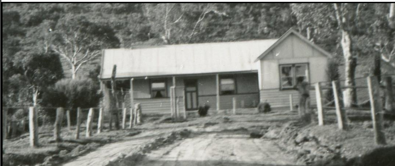
The McKinlay house c1940s, sitting at the foot of Mt Moon. It was built by Eric with the help of his father Harry, with the extensions on the right (sitting room & kitchen) added following the initial construction.
